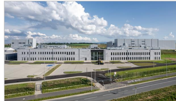
Commissioning of Umicore's new cathode materials plant in Nysa, Poland
